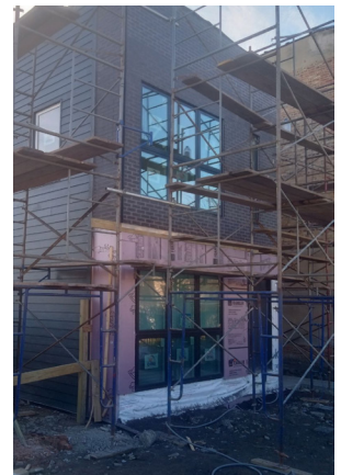
Home site, November 2023
