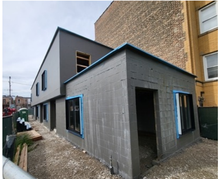
PSH Site B under construction in July 2023
